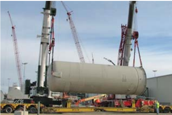
Cranes prepare to erect the nitrogen storage vessel after its 1,800 mile tour from Idaho to Kentucky.
