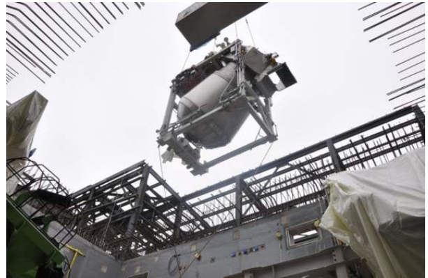
An Energetics Batch Hydrolyzer (EBH) is lowered into the Munitions Demilitarization Building (MDB) to process the energetic portions of munitions.
