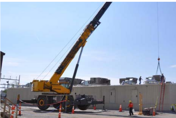
The modular laboratory buildings have arrived at the BGCAPP site and are being placed.
