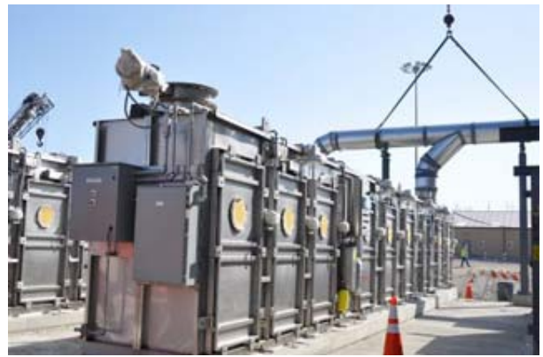
Carbon filter banks serve as the last stage of the cascading air filtration system on the MDB.
