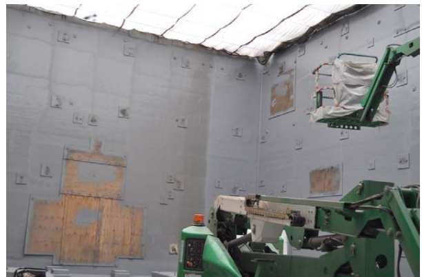
Protective coatings are applied to the MDB concrete to prevent any migration of chemicals from the building and make any necessary cleanup easier for the workers.
